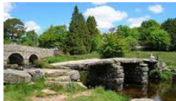
The Old Clapper Bridge, Postbridge
