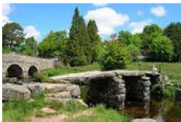
The Old Clapper Bridge, Postbridge
