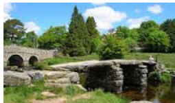
The Old Clapper Bridge, Postbridge
