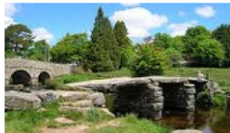
The Old Clapper Bridge, Postbridge
