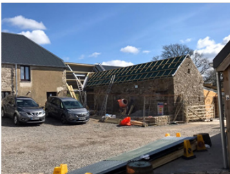
The old Corner Barn, reinstated and extended. The Shippen receives a new floor, roof and some heating.
