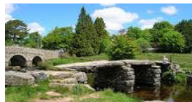
The Old Clapper Bridge, Postbridge
