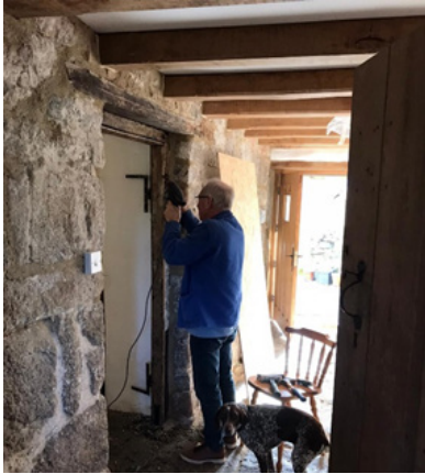
Dave Adams stripping the door frame
