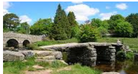
The Old Clapper Bridge, Postbridge
