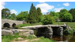
The Old Clapper Bridge, Postbridge
