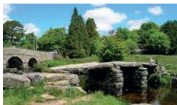
The Old Clapper Bridge, Postbridge
