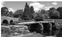
The Old Clapper Bridge, Postbridge
