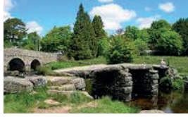
The Old Clapper Bridge, Postbridge
