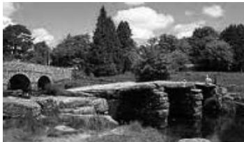
The Old Clapper Bridge, Postbridge
