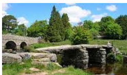
The Old Clapper Bridge, Postbridge
