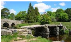
The Old Clapper Bridge, Postbridge
