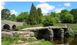
The Old Clapper Bridge, Postbridge
