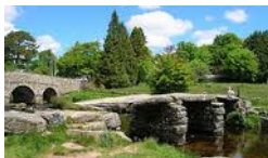
The Old Clapper Bridge, Postbridge
