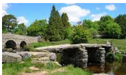
The Old Clapper Bridge, Postbridge
